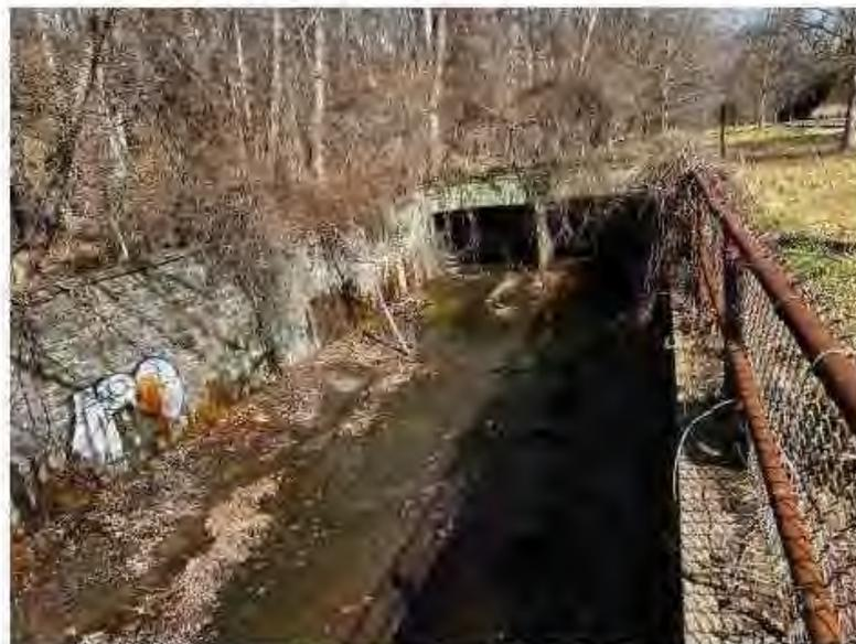
**Photo 2:** Former single-gate outfall was converted to a double-gate outfall in 1957 (Traceris, 2022).
