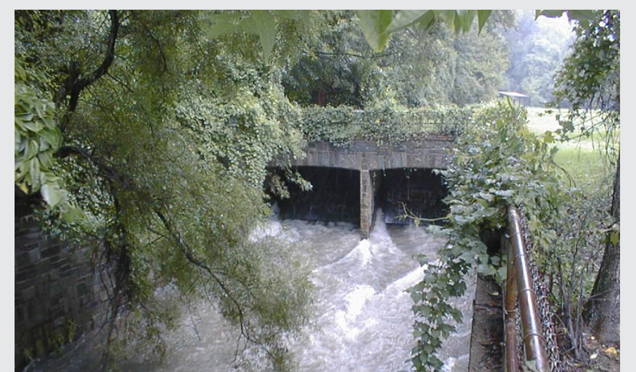
Combined sewer overflow discharge to the Piney Branch.
