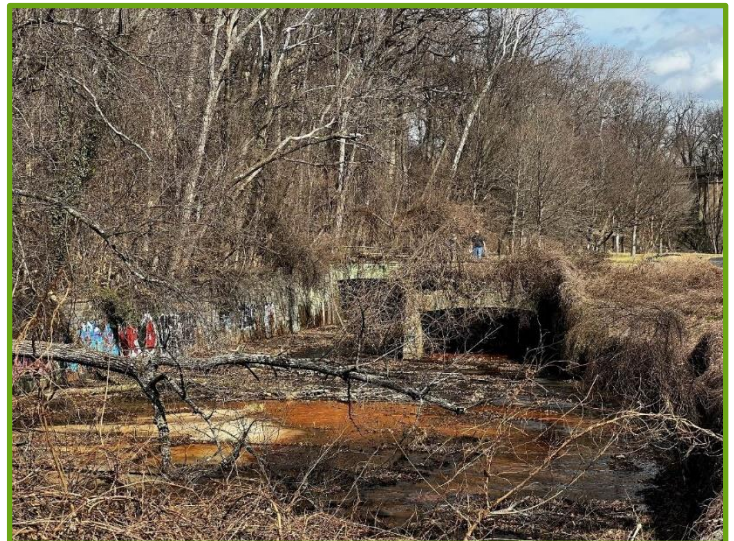
Upstream view of the existing CSO 049 outfall
