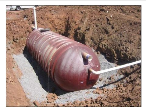
Figure 7-7. Irrigation cistern at Wetland Studies and Solutions, Inc. (overflow to rain garden). (Source: Wetland Studies and Solutions, Inc.)
