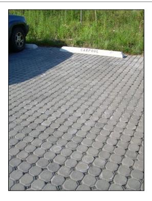
Figure 3-14. Pervious pavers in parking area. (Source: Wetland Studies and Solutions, Inc.)
