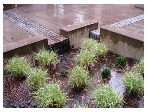
Figure 2-7. Bioretention planter in an urban courtyard. (Source: Portland SWM Manual)
