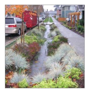
Figure 5-1. Vegetated swale (bioswale) in High Point, WA. (Source: American Planning Association – Washington Chapter)
