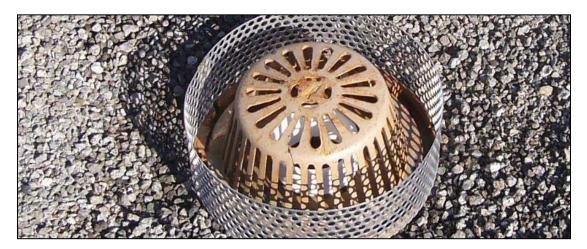
Figure 8-3. Strainers or screens help prevent debris from clogging roof drains. (Source: New York City Department of Environmental Protection)
