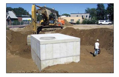
Figure 7-4. Multiple underground cisterns in series. (Source: LID Manual for Michigan)
