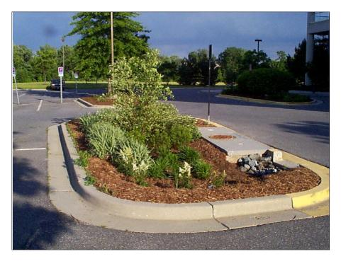
Figure 2-8. Bioretention in a parking lot island. (Source: NCDENR Stormwater BMP Manual)
