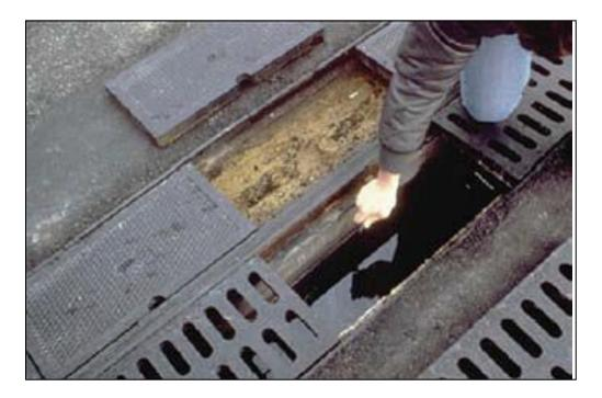
Figure 9-8. Access for maintenance of perimeter filter system. (Source: LID Manual for Michigan )
