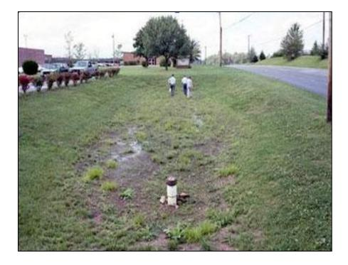
Figure 9-9. Sand filter application with vegetation. (Source: Virginia DCR Stormwater Design Manual)
