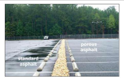
Figure 3-12. Porous and conventional asphalt. (Source: LID Manual for Michigan)
