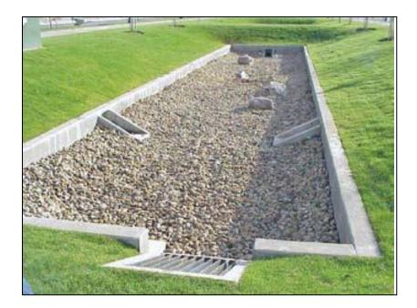
Figure 9-1. Surface filter system. (Source: Portland SWM Manual)
