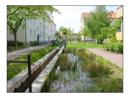
Figure 5-7. Wet swale and controlled canal in Champaign, IL. (Source: University of Illinois, Department of Urban and Regional Planning)
