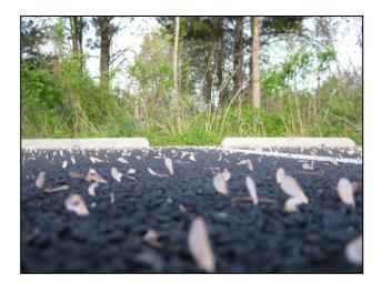
Figure 3-6. Red maple seeds lodged in pores of permeable asphalt. (Source: Wetland Studies and Solutions, Inc.)
