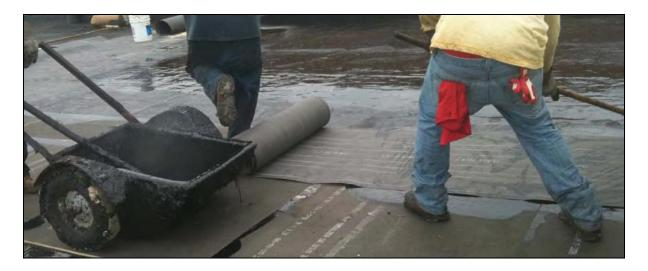
Figure 8-7. Installation of a waterproof membrane during blue roof construction. (Source: New York City Department of Environmental Protection)
