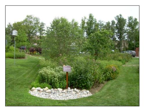
Figure 2-9. Bioretention facility treating parking lot and rooftop. (Source: Wetland Studies and Solutions, Inc.)
