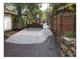
Figure 3-2. Constructing a green alley in Chicago. (Source: City of Chicago)
