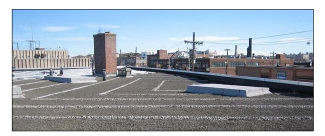
Figure 8-2. Check dams installed to control flow on sloped portion of roof, Brooklyn, NY. (Source: New York City Department of Environmental Protection)
