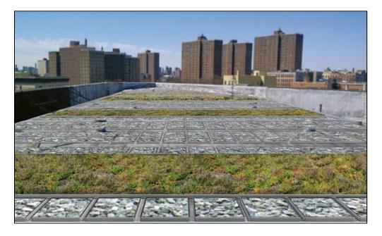
Figure 8-6. Blue roof installed in combination with green roof, New York, NY. (Source: New York Department of Environmental Protection/Hazen and Sawyer)
