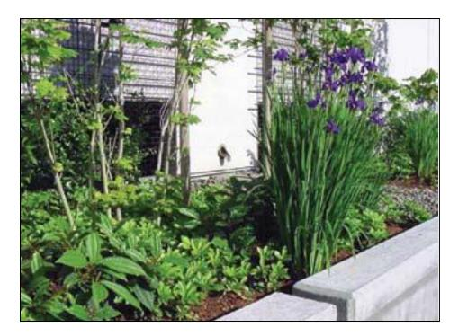
Figure 2-5. Typical bioretention planter box adjacent to a building. (Source: City of Portland SWM Manual)
