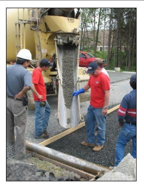
Figure 3-5. Placement of pervious concrete. (Source: Wetland Studies and Solutions, Inc.)
