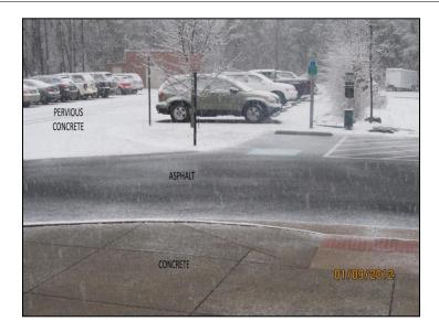
Figure 3-7. Pervious concrete parking lot in snow – note coverage compared to conventional paving materials. (Source: Wetland Studies and Solutions, Inc.)
