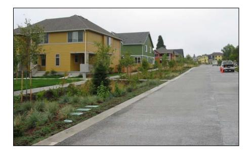
Figure 3-13. Pervious concrete residential street. (Source: City of Seattle Stormwater Manual)
