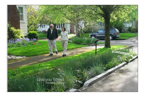
Figure 2-1. Curb-extension bioretention facility (Source: UACDC LID Design Manual for Urban Areas)
