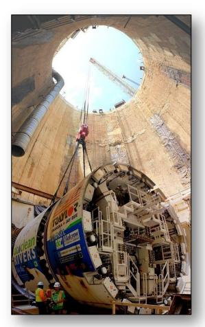
"Lady Bird" Tunnel Boring Machine for the Blue Plains Tunnel
