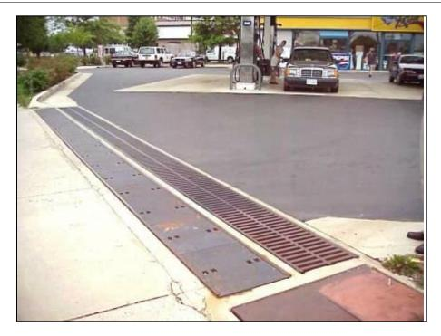
Figure 9-7. Perimeter filter system. (Source: Chesapeake Bay Stormwater Network)
