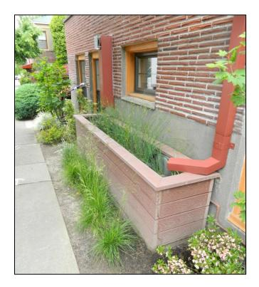
Figure 3-14. Downspout disconnect to stormwater planter. (Source: U.S. EPA)
