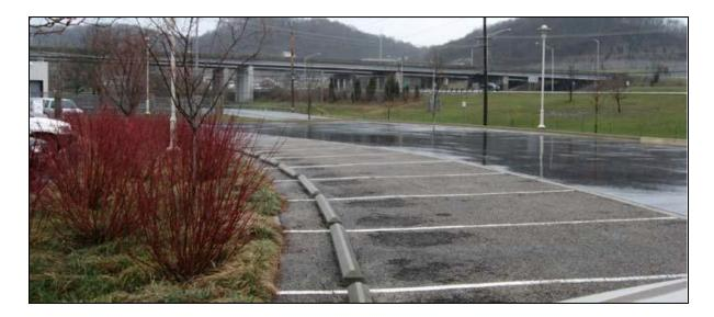
Figure 3-9. Pervious concrete in parking lot stalls. (Source: SWM Handbook for Northern Kentucky)
