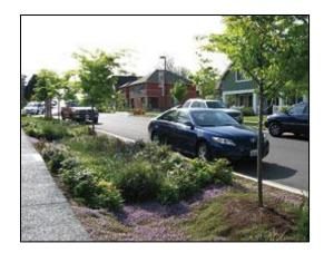
Figure 3-11. Street swale and pervious pavement in Seattle neighborhood. (Source: Washington State University)
