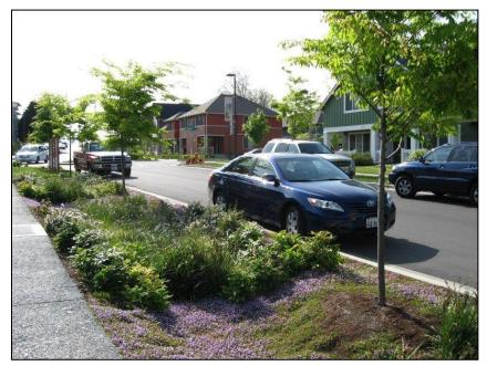
Figure 5-2. New residential street uses a vegetated swale to capture runoff. (Source: U.S. EPA)
