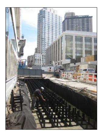
Figure 4-5. Installation of Silva Cells at Lincoln Center (Source: Deep Root Partners L.P.)
