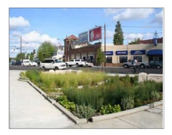
Figure 2-2. Small bioretention facility retrofitted in a busy urban setting. (Source: Nevue Ngan Associates)
