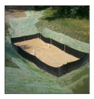
Figure 9-2. Surface sand filter during construction (Source: Chesapeake Bay Stormwater Network)
