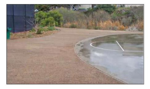
Figure 3-11. Colored pervious concrete. (Source: LID Manual for Michigan)
