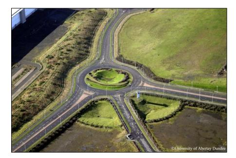
Figure 3-18. Green detention basin at DEX roundabout. (Source: University of Abertay Dundee)
