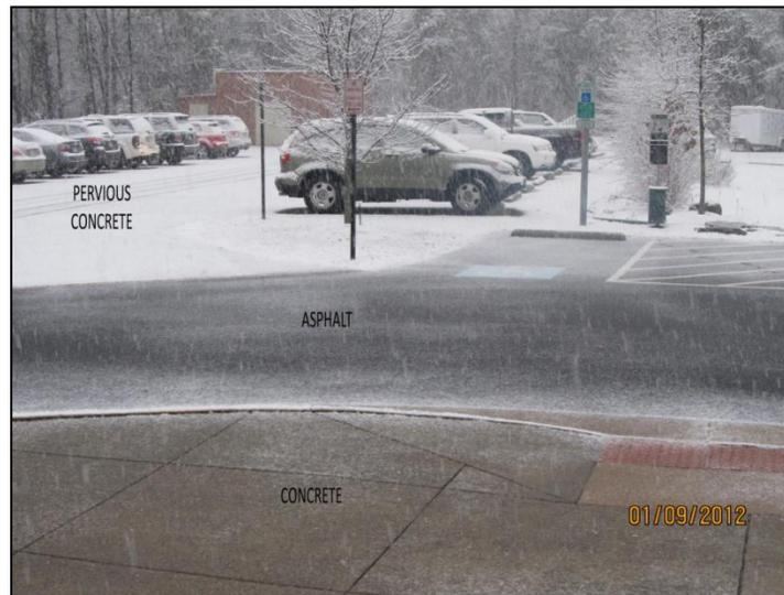
**Figure 3-7. Pervious concrete parking lot in snow – note coverage compared to conventional paving materials.
