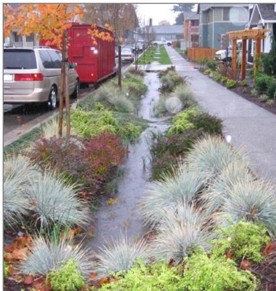
**Figure 5-1. Vegetated swale (bioswale) in High Point, WA.
