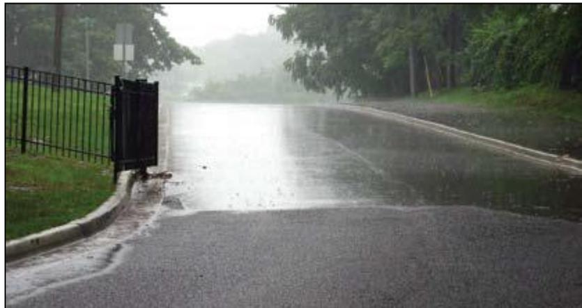
**Figure 3-2. Run-on from traditional asphalt pavement.
