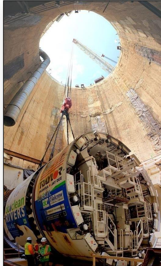
“Lady Bird” Tunnel Boring Machine for the Blue Plains Tunnel
