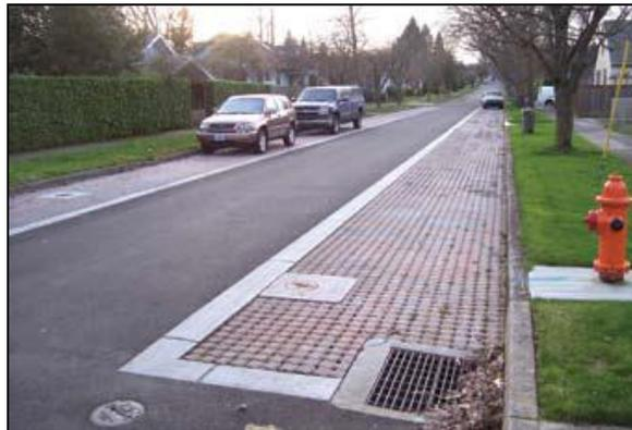
**Figure 3-1. Pervious paver shoulders along a residential street
