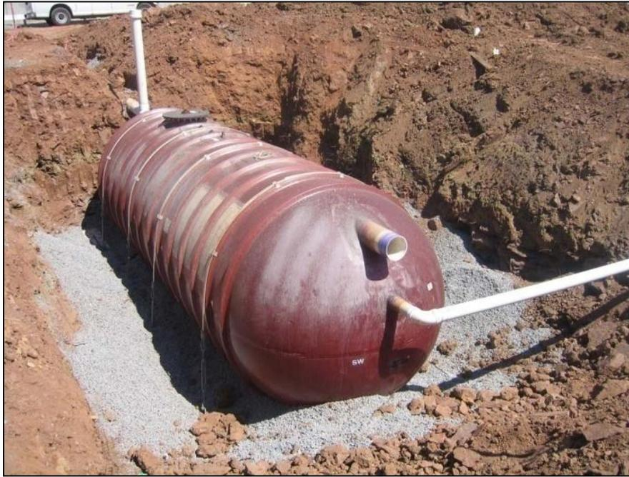
**Figure 7-7. Irrigation cistern at Wetland Studies and Solutions, Inc. (overflow to rain garden).
