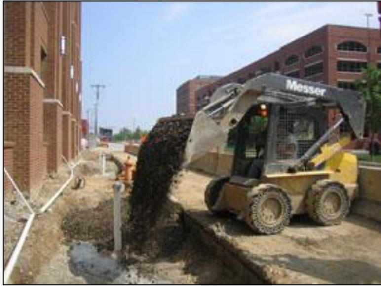
**Figure 4-7. Structural soil adjacent to a building.**
