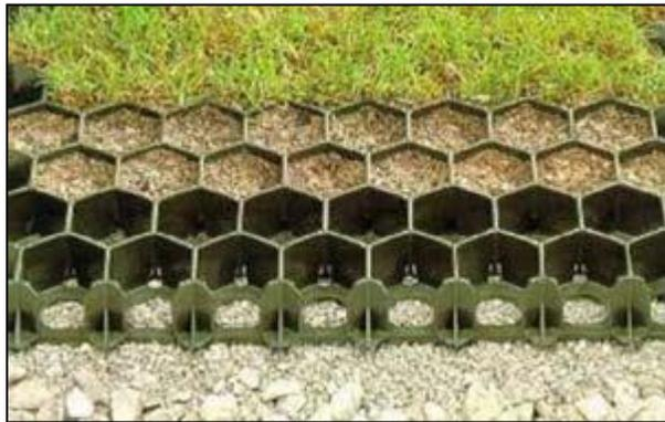
**Figure 3-8. Reinforced grid system.**
