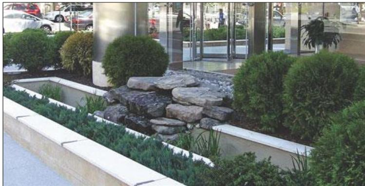
**Figure 2-3. Bioretention planter box in Washington, D.C.**
