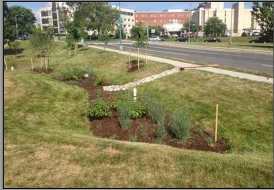
**DC Water Bioretention Facility at Irving St NW**
