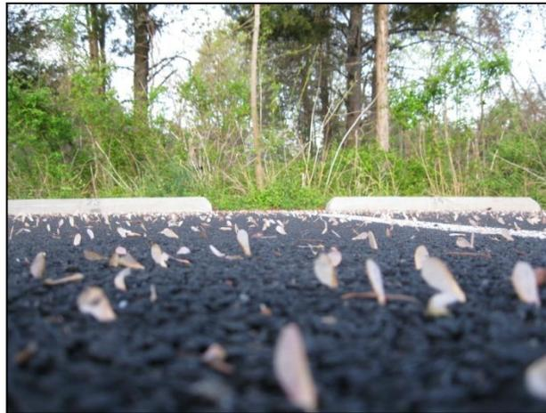
**Figure 3-6. Red maple seeds lodged in pores of permeable asphalt.
