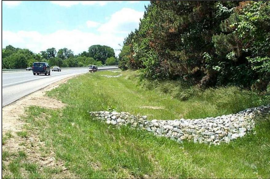
**Figure 5-8. Vegetated swale with check dams.
