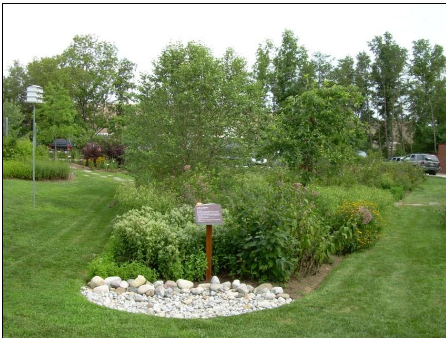
**Figure 2-9. Bioretention facility treating parking lot and rooftop.**
