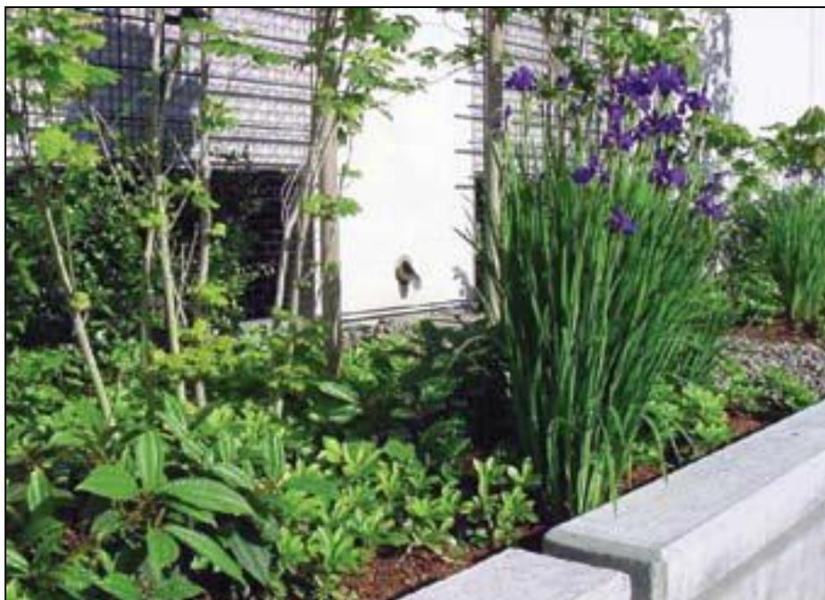
Figure 2-5. Typical bioretention planter box adjacent to a building.
