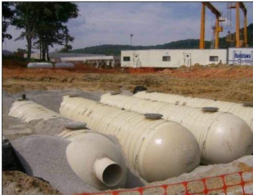
**Figure 7-3. Multiple underground cisterns in series.**
