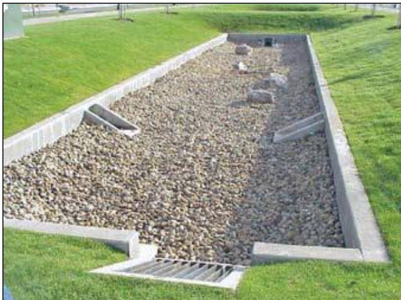
**Figure 9-1. Surface filter system.**
