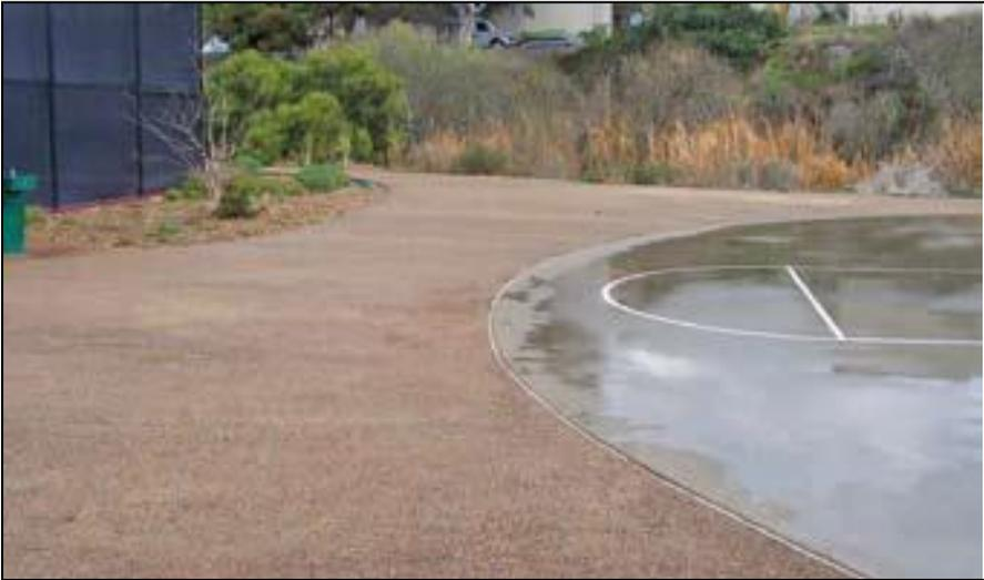
**Figure 3-11. Colored pervious concrete.
