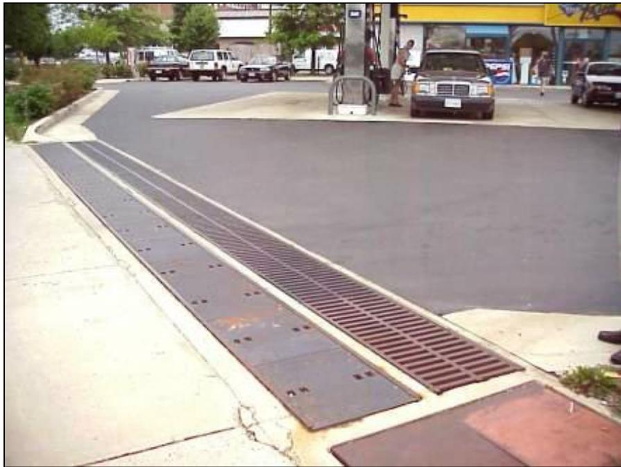
**Figure 9-7. Perimeter filter system.**
