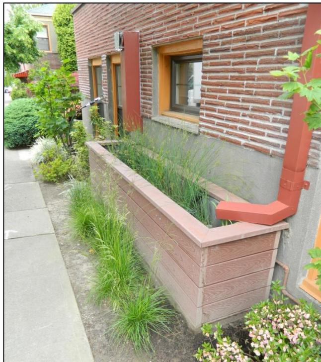
**Figure 3-14. Downspout disconnect to stormwater planter.**
