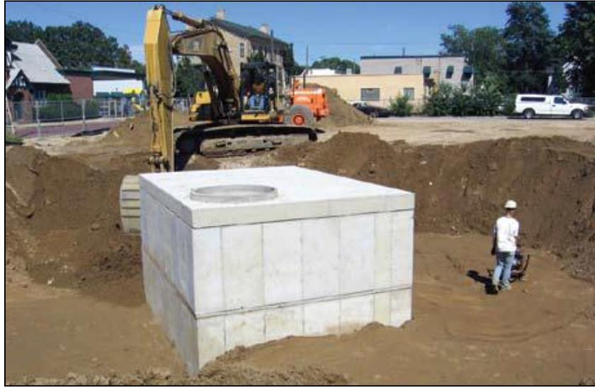
**Figure 7-4. Multiple underground cisterns in series.
