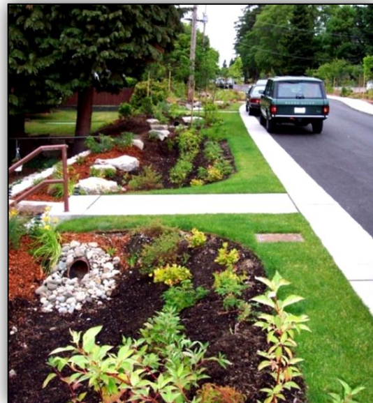
Bioretention Facility
