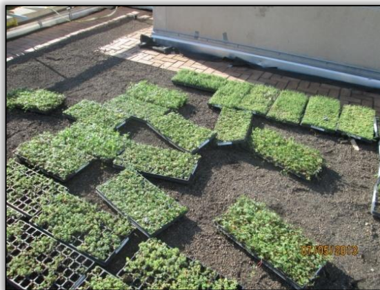
Green Roof During Construction at DC Water's East Side Pumping Station
