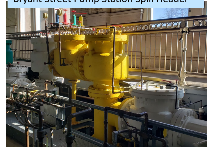
Bryant Street Pump Station Spill Header
