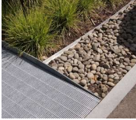
3) Grated Boardwalk Crossings
