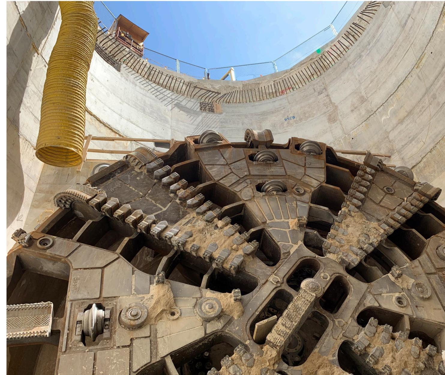
DC Water Clean Rivers Project – NEBT boring machine cutterhead.
