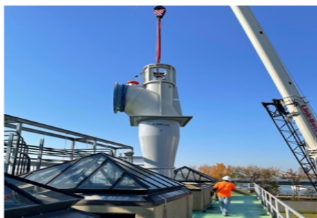
Blue Plains Filter Influent Pump Install
