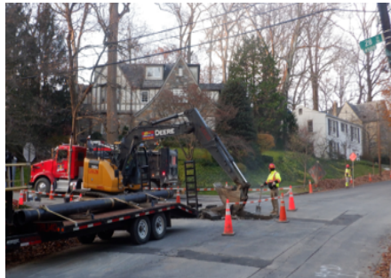
Small Diameter Water Main Repair
