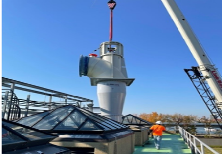
Blue Plains Filter Influent Pump Install
