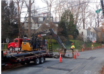
Small Diameter Water Main Repair
