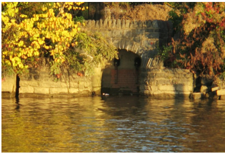
Combined Sewer Overflow Outfall
