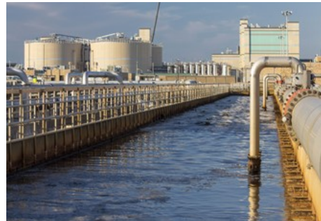
Secondary Sedimentation
