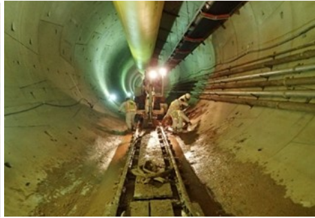
Northeast Boundary Tunnel
