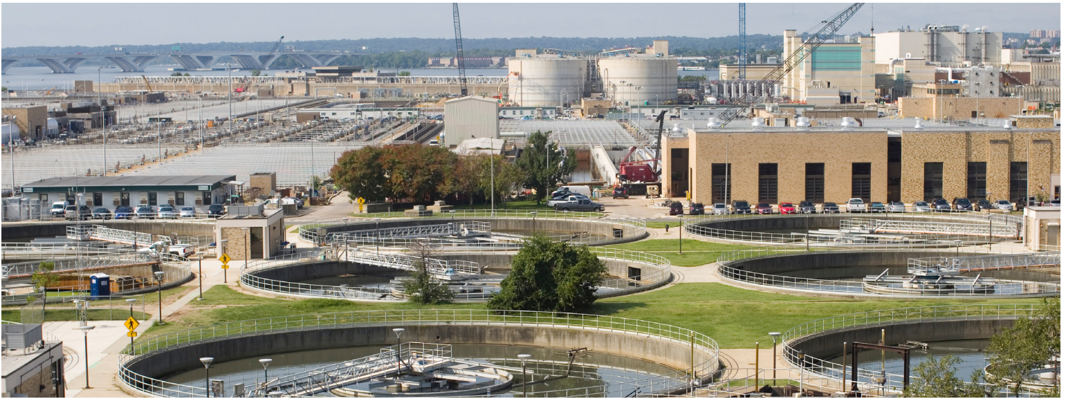
Blue Plains Advanced Wastewater Treatment Plant
