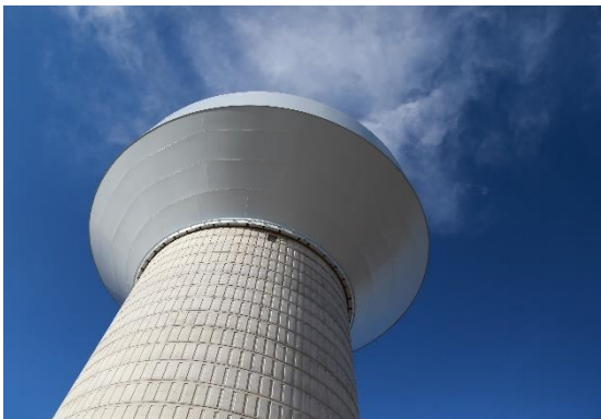
Saint Elizabeth Water Tower
