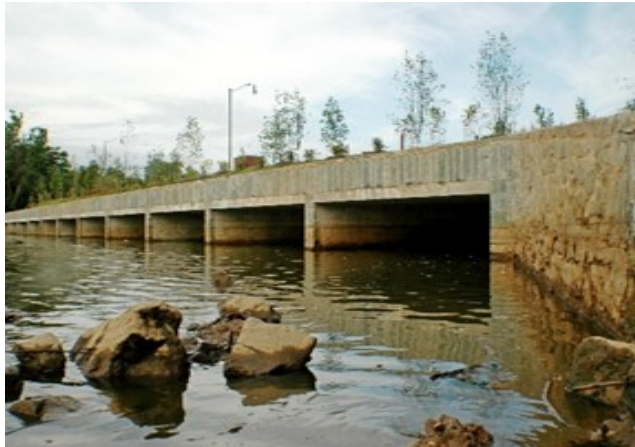
CSO 19 Overflow Facility
