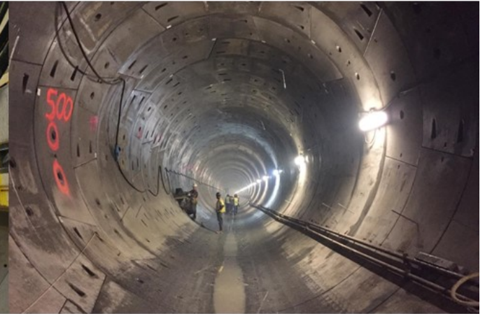
Combined Sewer Overflow
