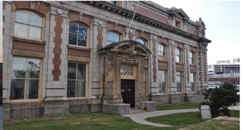
Main Pumping Station
