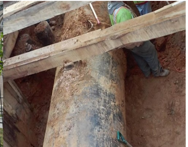
Large Valve Replacement
