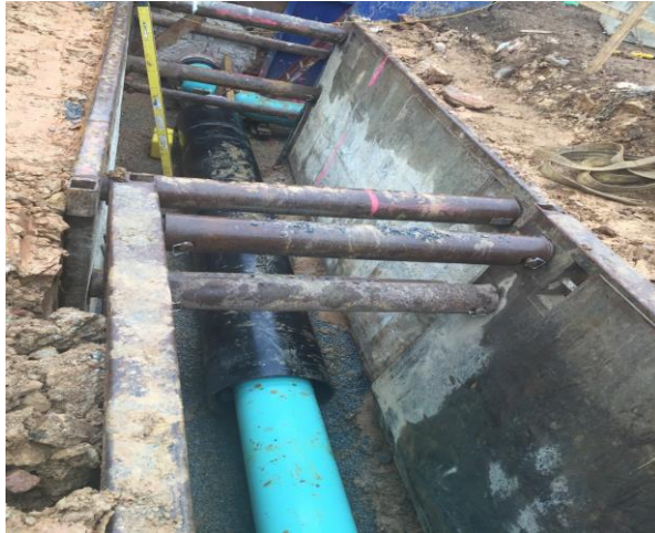
Work on Sewer Laterals
