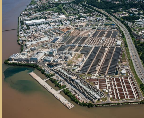
Blue Plains Advanced Wastewater Treatment Plant
