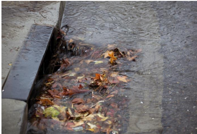
City Street Catch Basin
