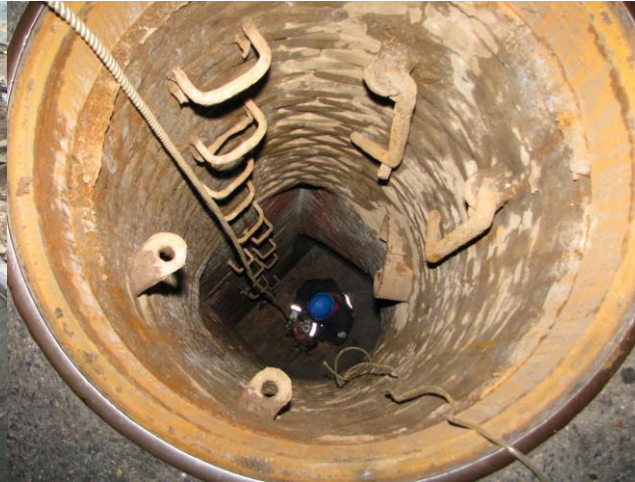
Sewer Inspection Work
