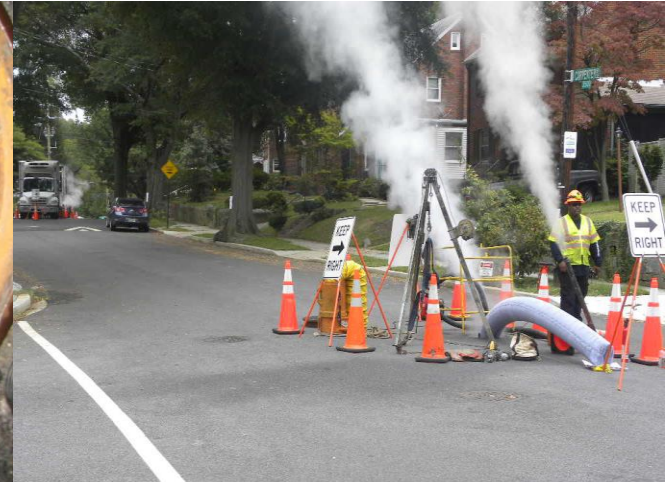
Sewer Rehabilitation - CIPP
