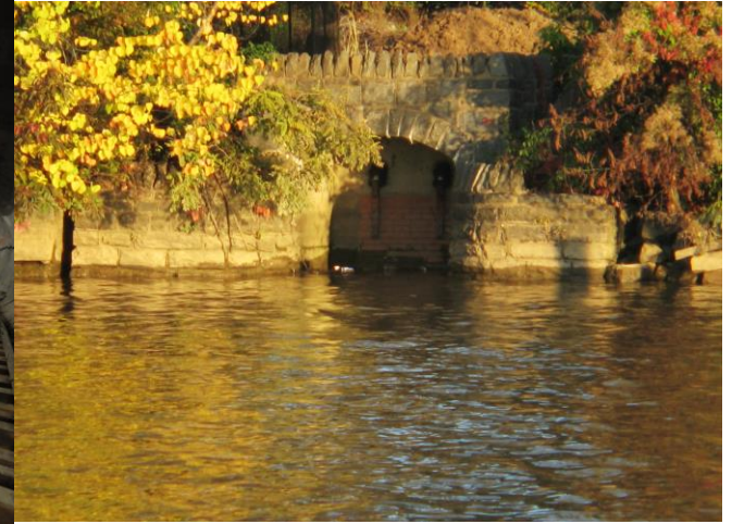
Combined Sewer Overflow Outfall
