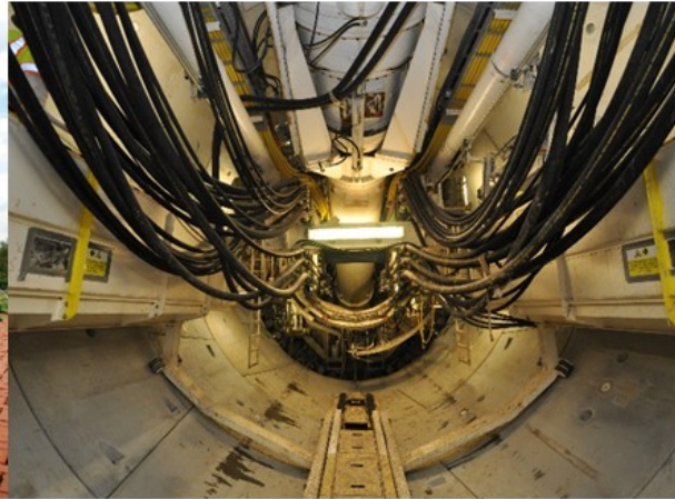
Tunnel Boring Machine
