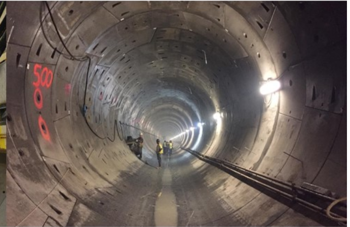
Combined Sewer Overflow
