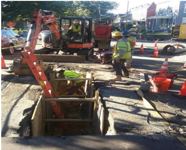
Small Diameter Water Main Replacement
