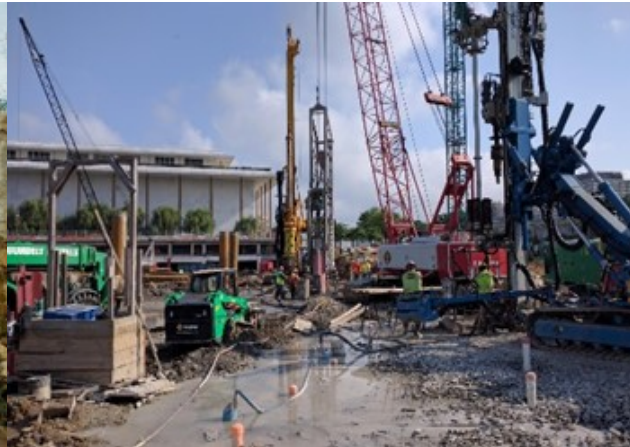
CSO 21 Diversion Facilities
