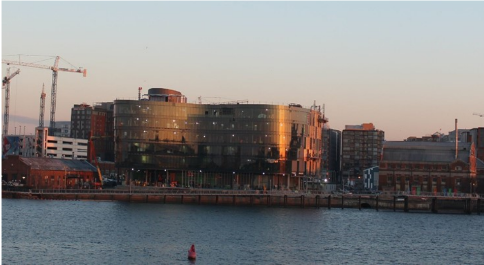
New Headquarters Building (HQO)
