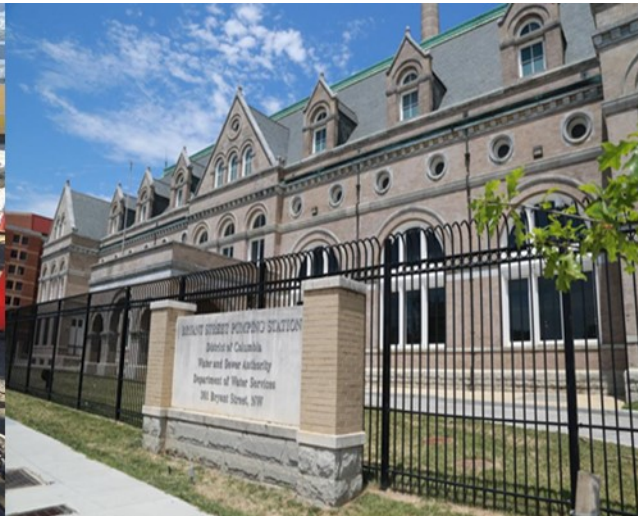
Bryant Street Pumping Station
