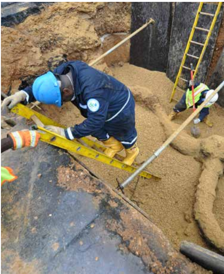
Water main replacement
