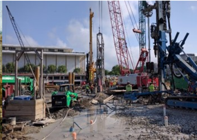
CSO 21 Diversion Facilities
