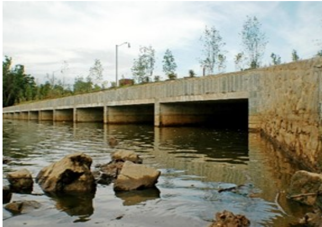
CSO 19 Overflow Facility
