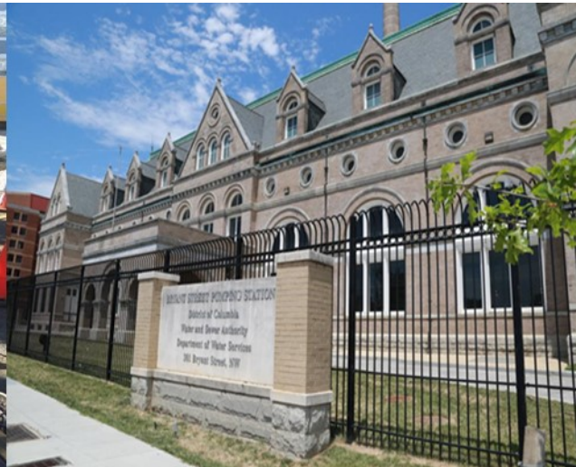
Bryant Street Pumping Station
