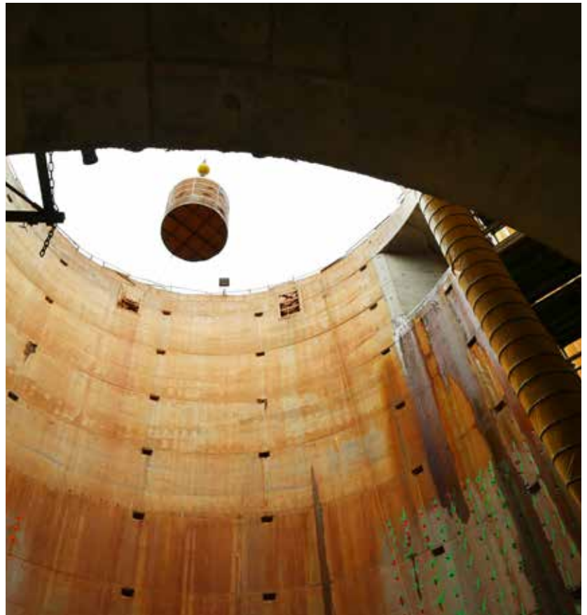
Clean Rivers Anacostia River tunnel shaft
