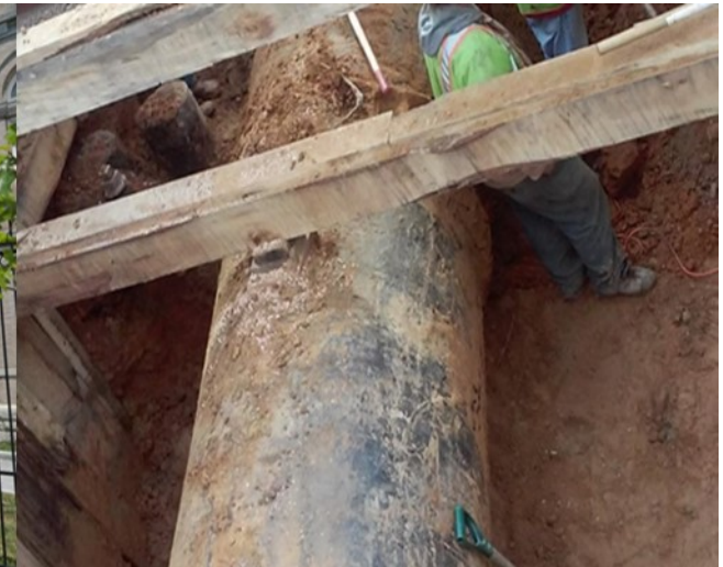
Large Valve Replacement
