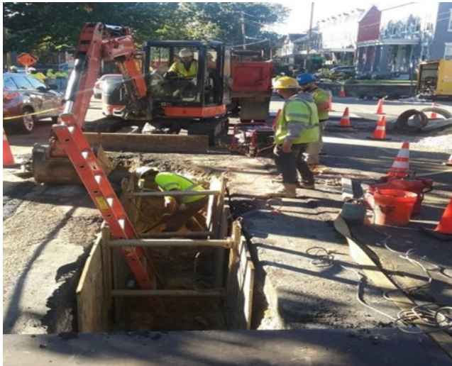
Small Diameter Water Main Replacement
