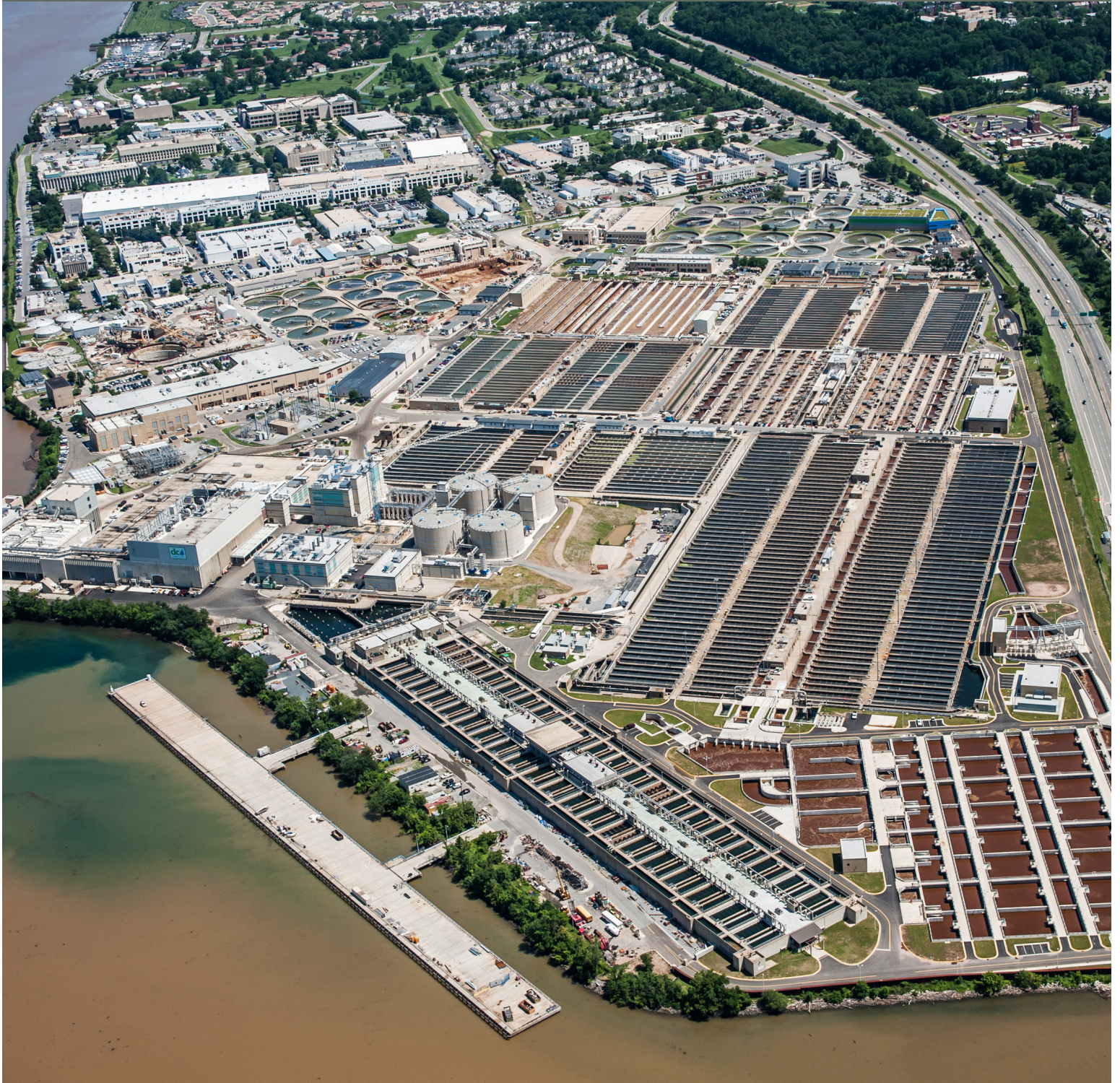
Blue Plains Advanced Wastewater Treatment Plant
