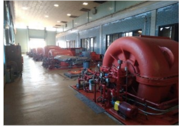
Photo A.9: Blue Plains AWWTP – nitrification blowers (PEER photo)
