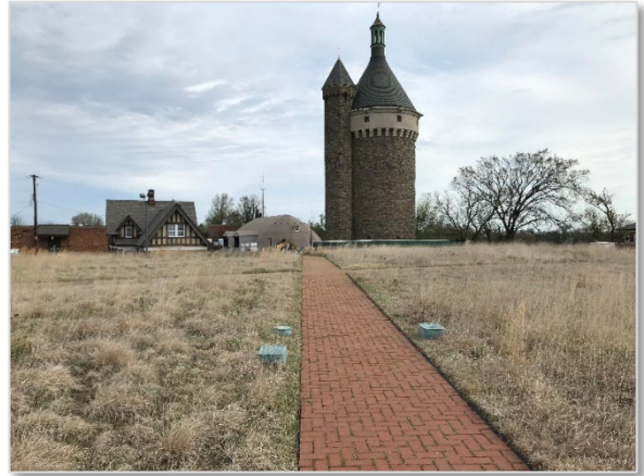
Photo A.4: Fort Reno Covered Reservoir – green roof plantings and permeable walk pavers (PEER photo)
