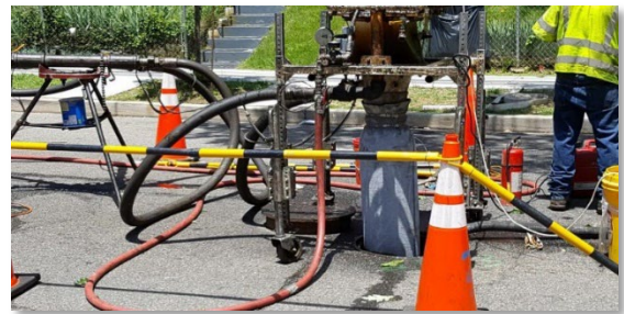
Photo 5-5: Sewer Rehabilitation (DC Water photo)
