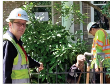
Photo 7-6: Lead Service Line being replaced (PEER photo)
