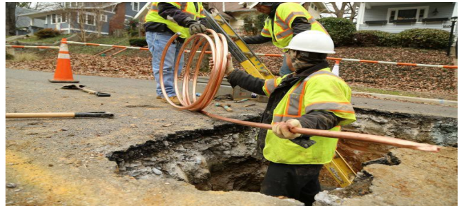
Photo 7-5: Replacing Lead Service Lines with Copper (DC Water photo)
