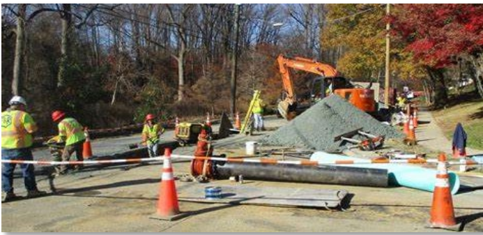
Photo 4-7: Small Diameter Water Main Replacement Program (DC Water photo)
