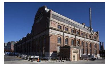
Photo 5-8: Main Pumping Station (Governing.com photo)
