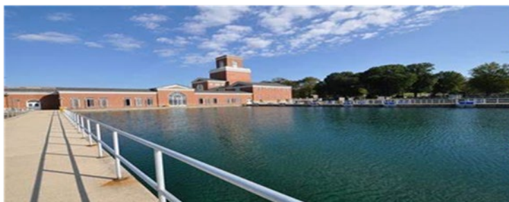
Photo 4-1: Dalecarlia Reservoir, Treatment Plant and Pumping Station (DC Water photo)
