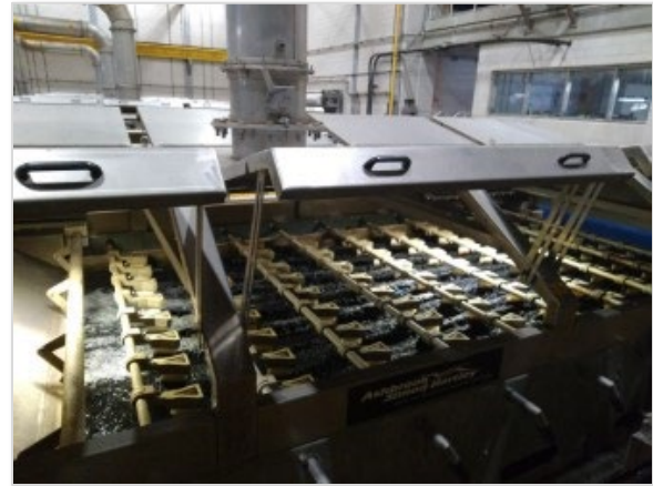
Photo A.10: Blue Plains AWWTP – belt filter press, gravity belt section (PEER photo)
