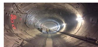
Photo 7-2: Northeast Boundary Tunnel (DC Water photo)
