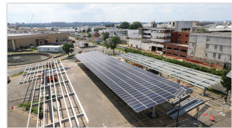
Photo 9-3: Solar Canopy Construction at Blue Plains AWWTP (DC Water photo)
