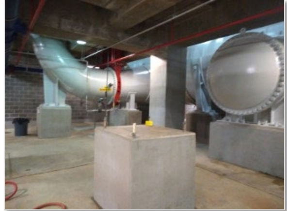
Photo A.13: Blue Plains AWWTP Stormwater Tunnel Pumping Station – pump suction header (PEER photo)
