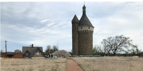
Photo 4-3: Fort Reno Pumping Station (PEER photo)
