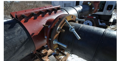
Photo 5-6: Potomac Interceptor (PI) Rehabilitation (DC Water photo)
