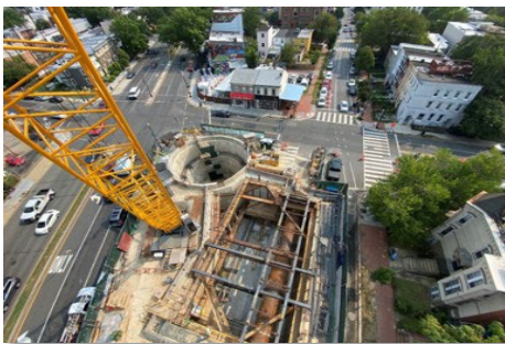
Photo 6-1: Clean Rivers Project Northeast Boundary Tunnel B Street (DC Water photo)
