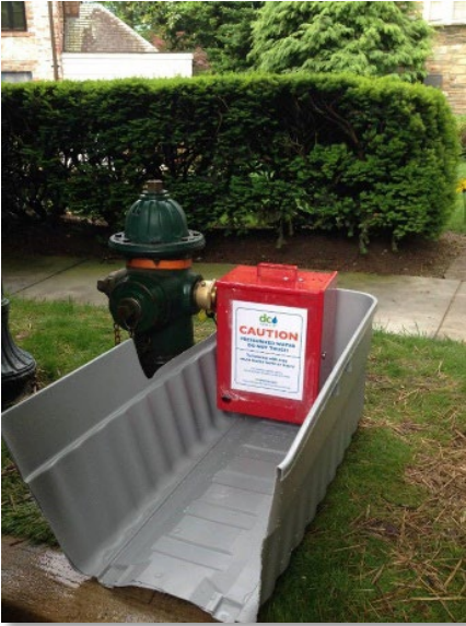
Photo 4-8: Automated Hydrant Flushing (DC Water photo)
