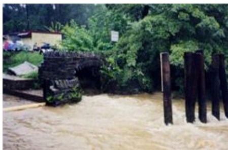
CSO Discharge to Anacostia River
