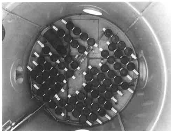
Reconfigured Aeration Pilot Diffusers for Fouling Mitigation Studies
