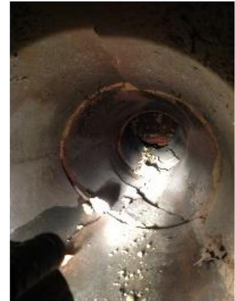
Vitrified Clay Pipe collapsed Small Dia. sewer
