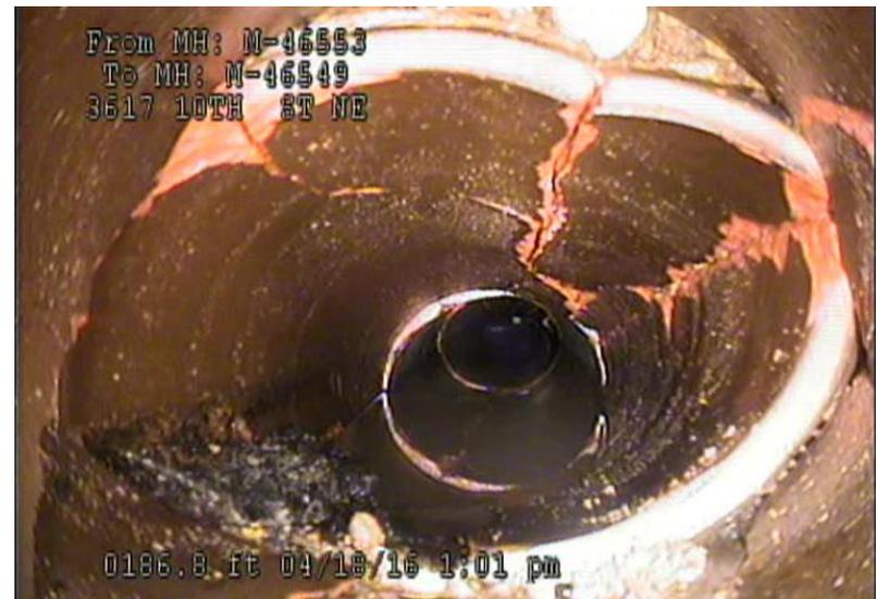
10<sup>th</sup> St at Otis St, NE (10" VCP, deformed, broken
