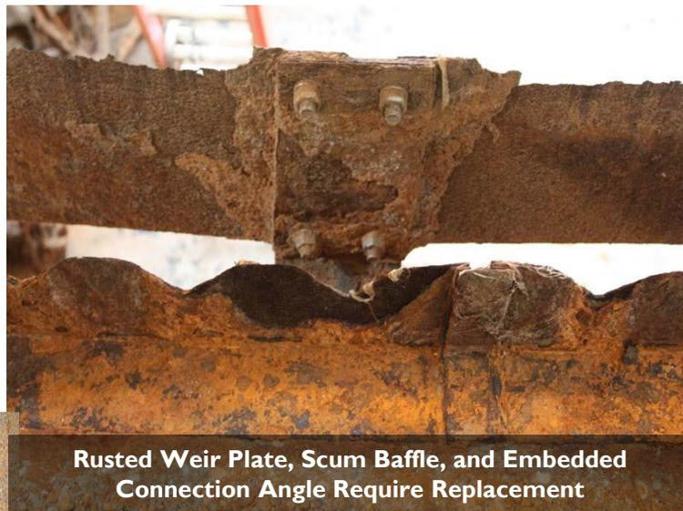
**Rusted Weir Plate, Scum Baffle, and Embedded Connection Angle Require Replacement**
