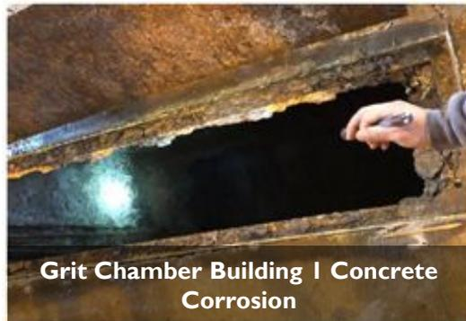
**Grit Chamber Building I Concrete Corrosion**
