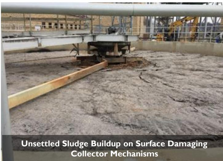
**Unsettled Sludge Buildup on Surface Damaging Collector Mechanisms**
