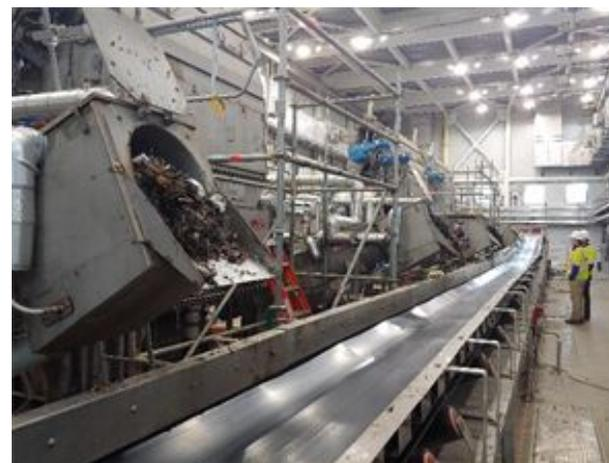
Trash and Debris Removed from CSO Captured by Tunnel at ECF Fine Screens
