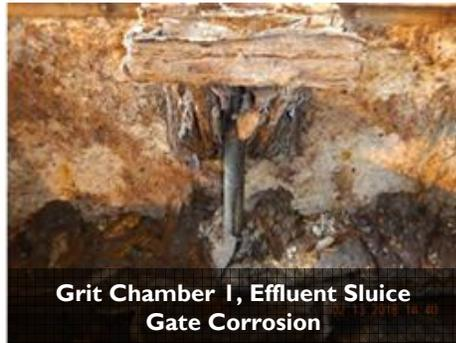
Grit Chamber 1, Effluent Sluice Gate Corrosion
