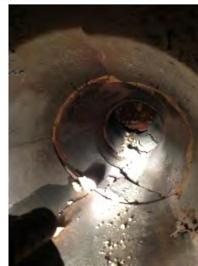
Vitrified Clay Pipe collapsed Small Dia. sewer
