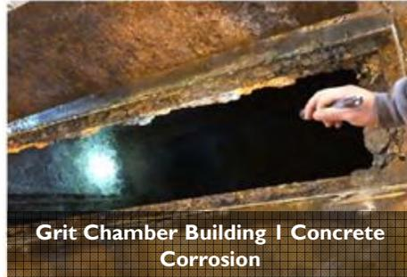
Grit Chamber Building 1 Concrete Corrosion
