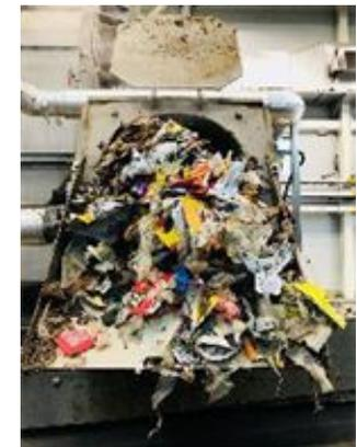
Trash removed by Fine Screenings at Wet Weather Treatment Facility
