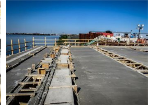
Overflow Structural Work
