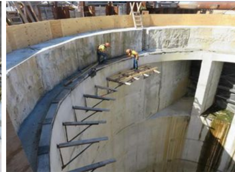
Drop Shaft Internals
