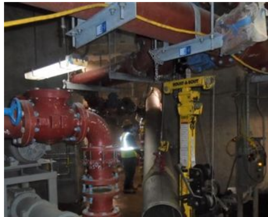
Blue Plains Gravity Thickener Upgrades
