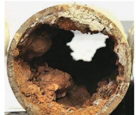
SDWM unlined Cast Iron pipe
