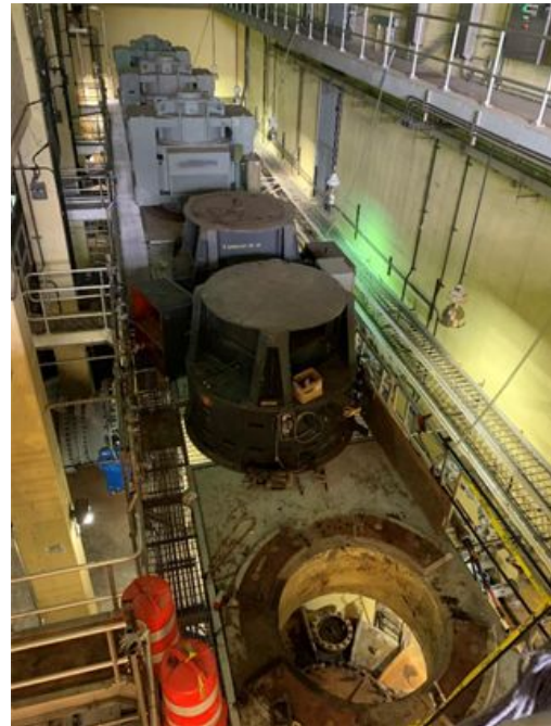
Potomac Pump Station Pump 5 Impeller removal
