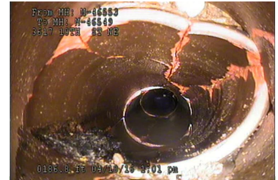
10th St at Otis St, NE (10" VCP, deformed, broken)
