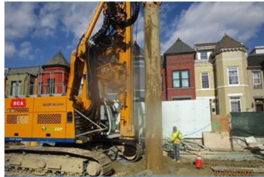
T Street - Soldier Pile Installation DCCR
