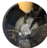
Northeast Boundary Tunnel
