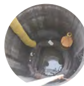
Mt. Olivet Shaft on Northeast Boundary Tunnel
