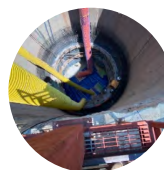
W Street Shaft on Northeast Boundary Tunnel
