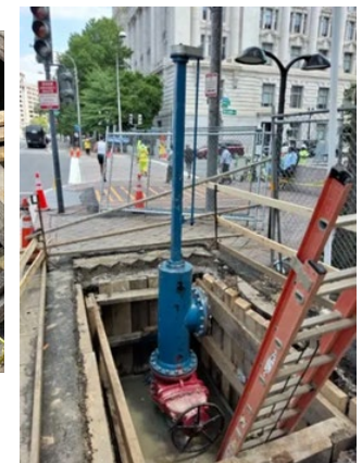
Line Stop Installation at 14th & Pennsylvania Ave NW, 07/23/2026
