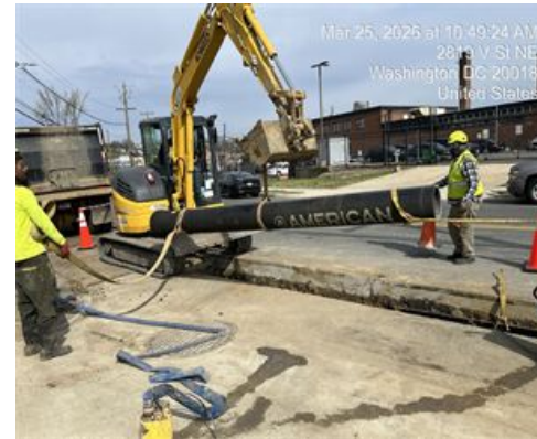
12" Water main installation on V St NE, 3/25/2026
