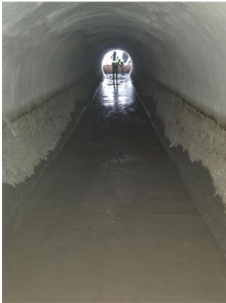
Paved invert prepared for slipline
