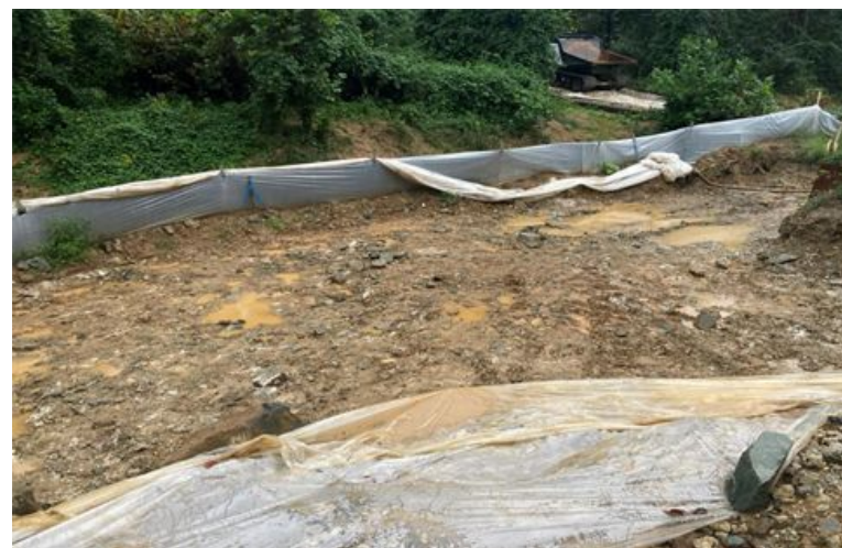
Cleanup of Soil Stockpile Area
