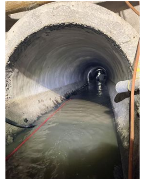
Geopolymer / bypass system condition
