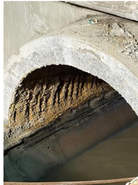
24/7 pump watch / bypass operations
