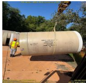
Pipe Delivery nearly 100%
