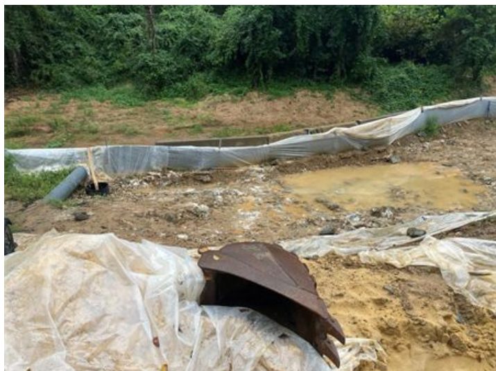
Canal / Rock Run rehabilitation area
