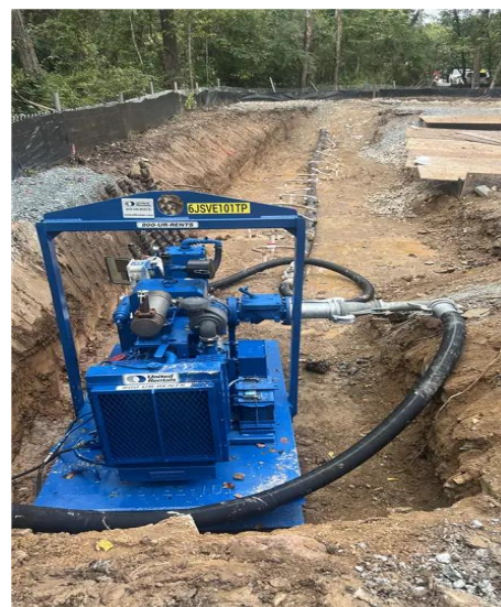
Push-pit excavation and installed wellpoints showing groundwater-control work.
