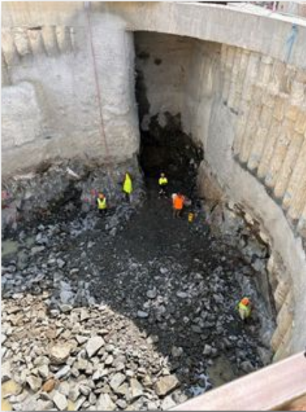
CSO 029: Shaft Rock Excavation
