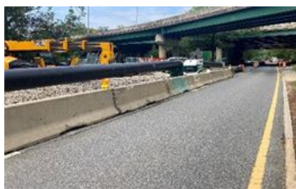
Bypass fusing staging area (and last trench TBD)
