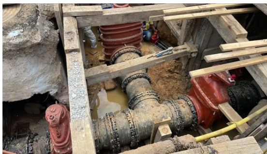
Installation of 30", 24" and a 20" Gate Valve at 17th & Gales ST NE, 06/03/2026
