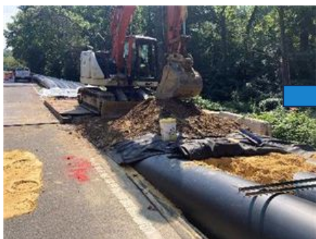
Bypass trench building 5 th location (before)
