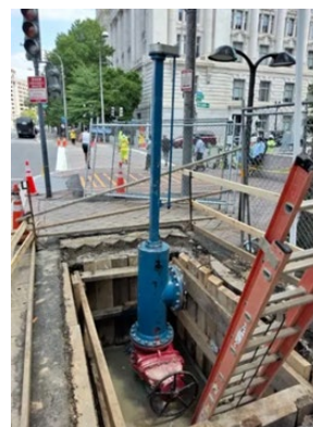
Line Stop Installation at 14th & Pennsylvania Ave
