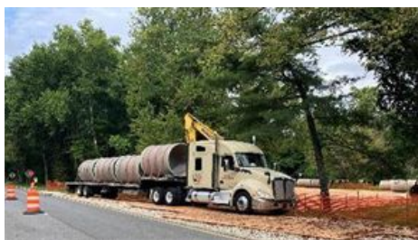
72-in Pipe Delivery Start
