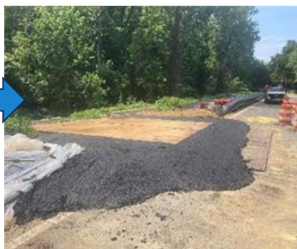
Bypass trench building 5 th location (after)
