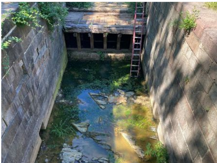
Lock 12 area after a rain event
