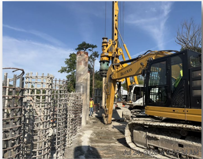
CSO 028: Secant Piles for Near Surface Structures
