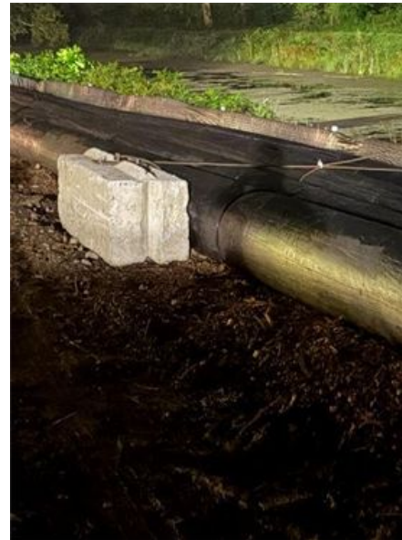
Bypass pipe secured with and blocks
