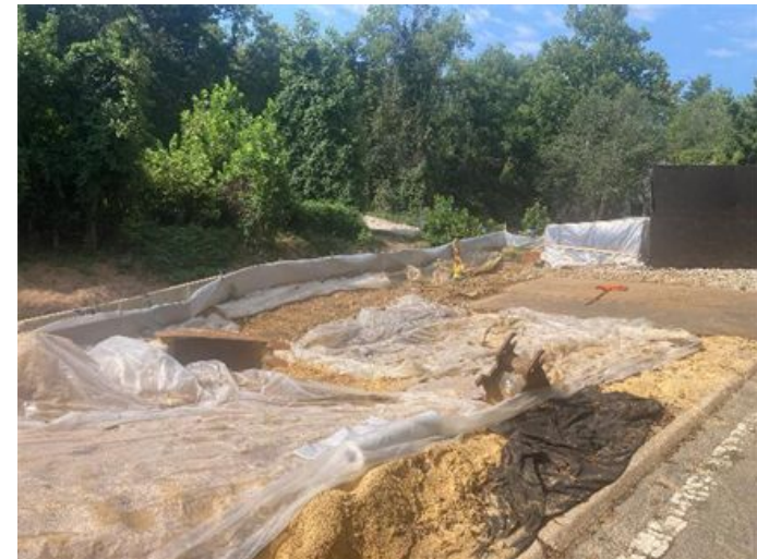
Cleanup of Soil Stockpile Area
