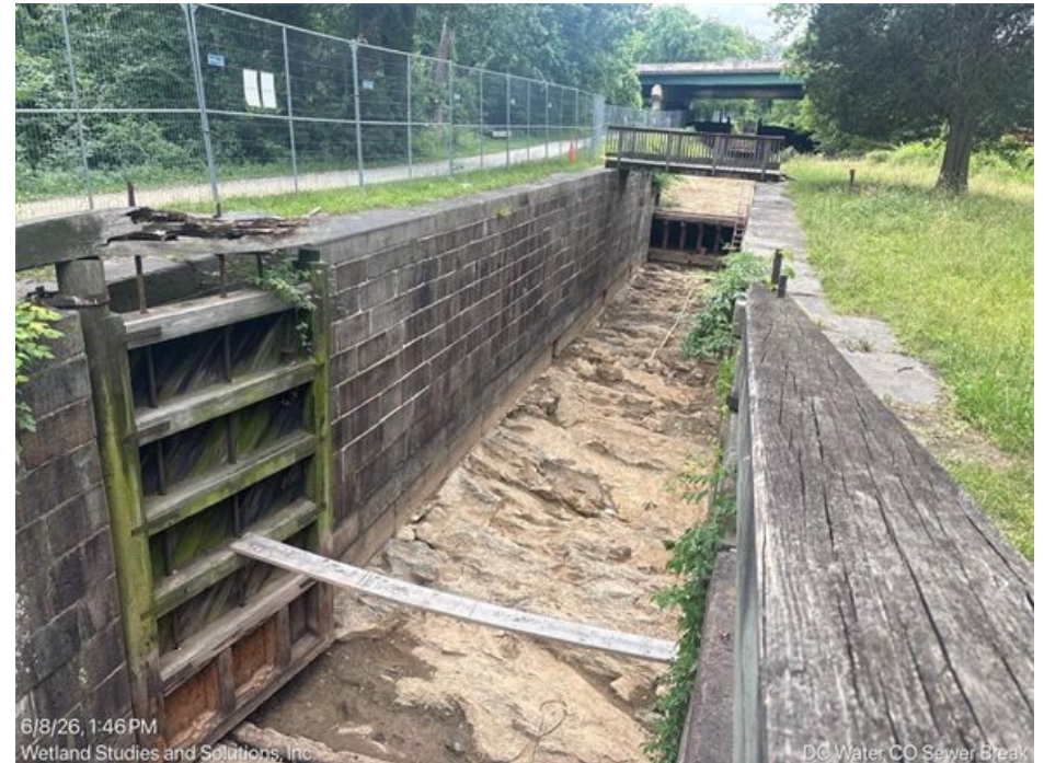
Lock 12 Cleaned to Bedrock (Area 4)
