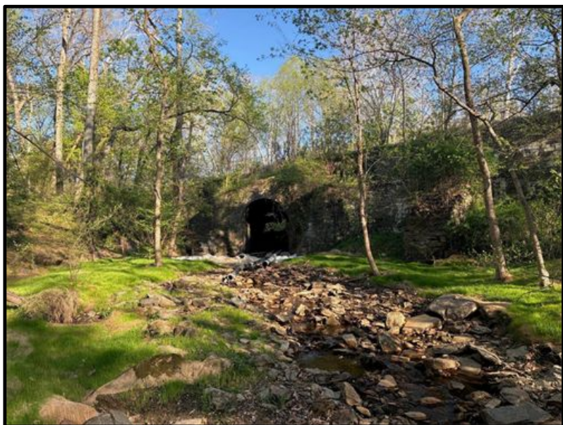
Area 2 Debris Removal and Temporary Stabilization Complete
