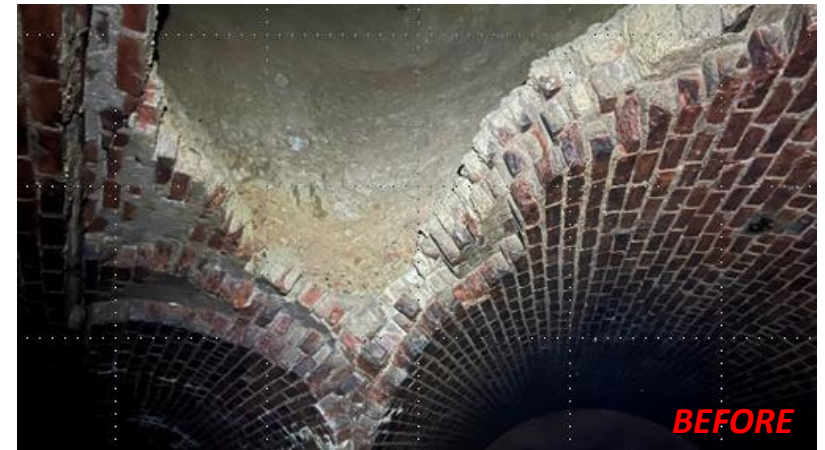
Northwest Boundary Trunk Sewer Repair – completed July 2025
