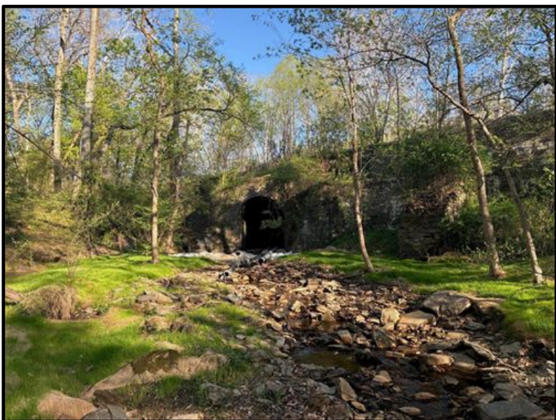
Area 2 Debris Removal and Temporary Stabilization Complete
