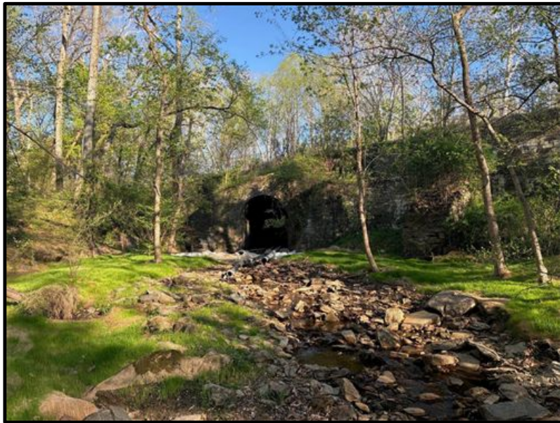
Area 2 Debris Removal and Temporary Stabilization Complete
