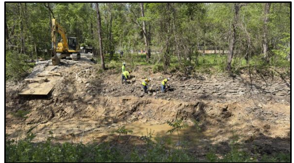
Restoration Work Within the Canal, Showing Access (Area 4)
