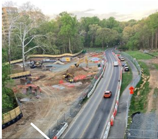
CSO 049: Construction of Relocated Piney Branch Parkway
