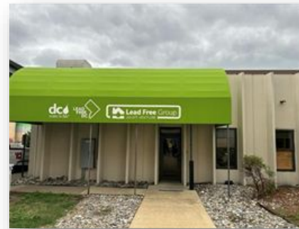
Renovation of existing 1970s building
