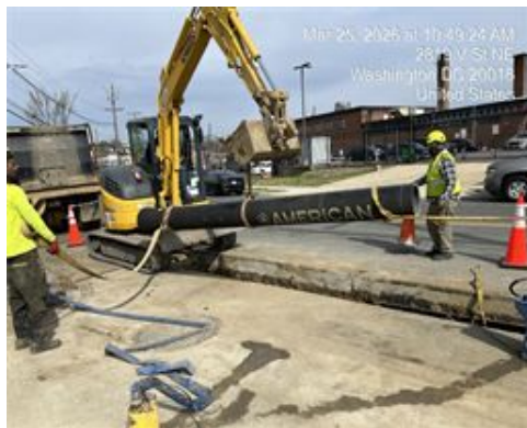
12" Water main installation on V St NE, 3/25/2026
