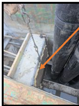
Bulkhead Removed
