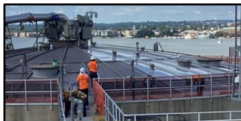
Digester Roof Repairs
