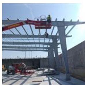
A Roof Covering the Structure
