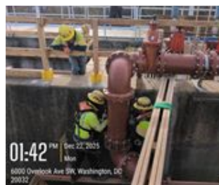
SWPS Piping Discharge Modifications
