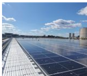
Solar Panel Installation & Wiring
