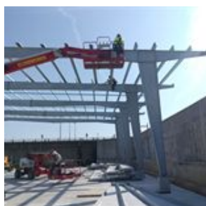
A Roof Covering the Structure
