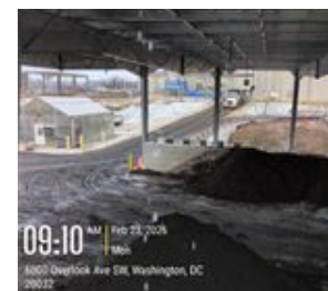
Biosolids Curing Pad in Use
