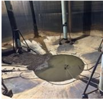
Digester 3 After Cleaning
