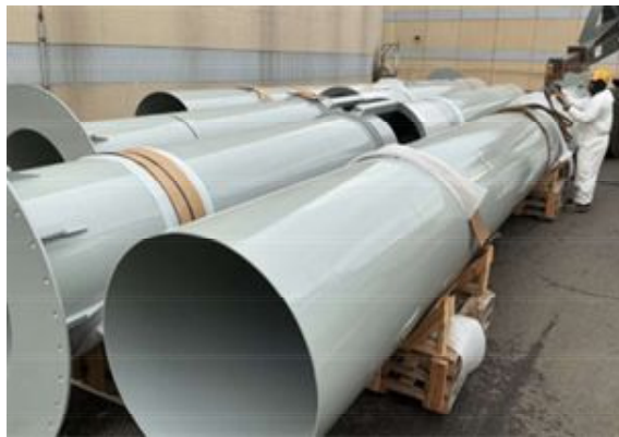
Rehabilitated draft tubes
