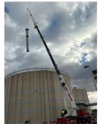
Contractor installing new draft tubes
