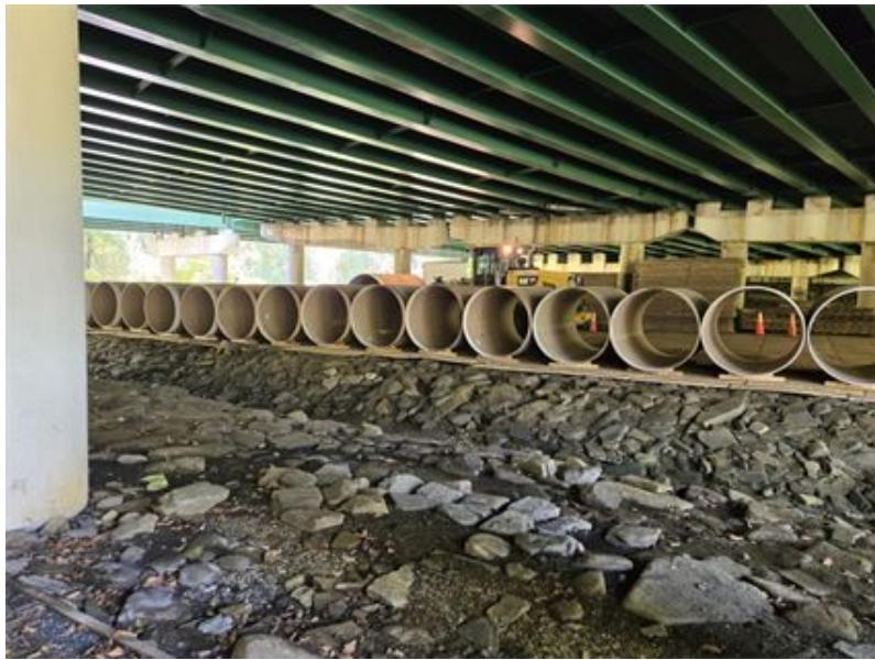
Eighty ten-feet sections of FRP were used to rehabilitate the PI.
