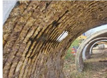
Corroded pipe crown and exposed reinforcing steel.
