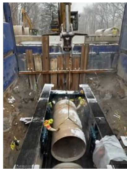
A 10-foot FRP section is lowered into the PI before being pushed into place.
