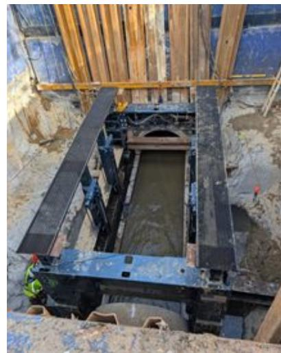
Pipe crown removed to create access for slip lining.
