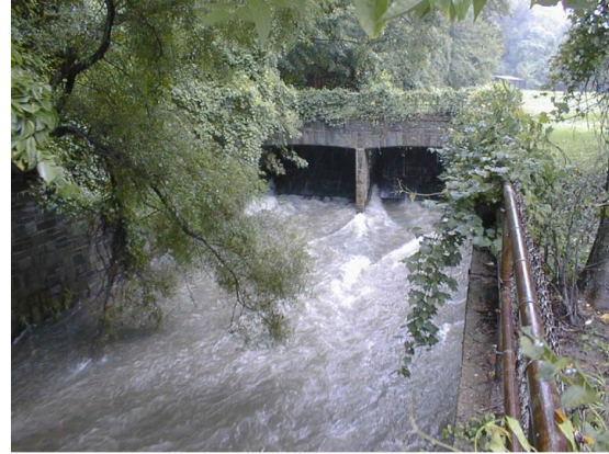
Projects like the Piney Branch tunnel will help manage combined sewer overflows in the District.
