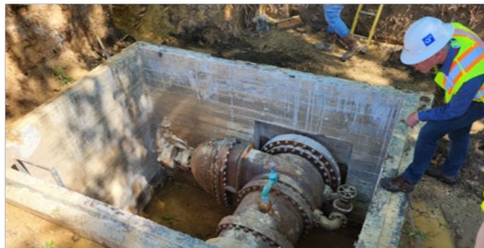
36" Valve Inspection at Fessenden Avenue NW
