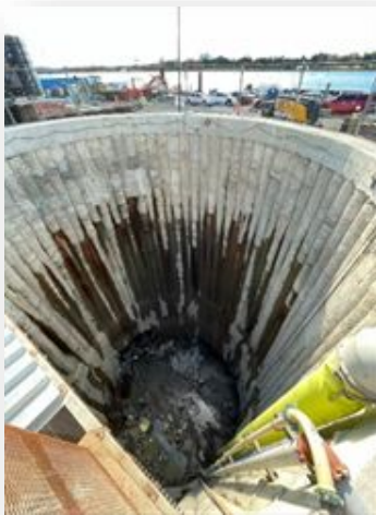
West Potomac Park: Starter Tunnels at Bottom of Shafts
