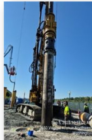
CSO 022: Secant Pile Construction for Shaft
