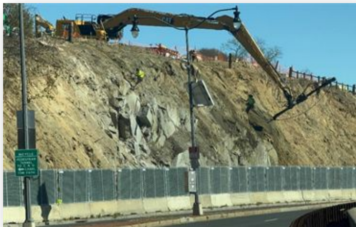
CSO 029: Slope Stabilization
