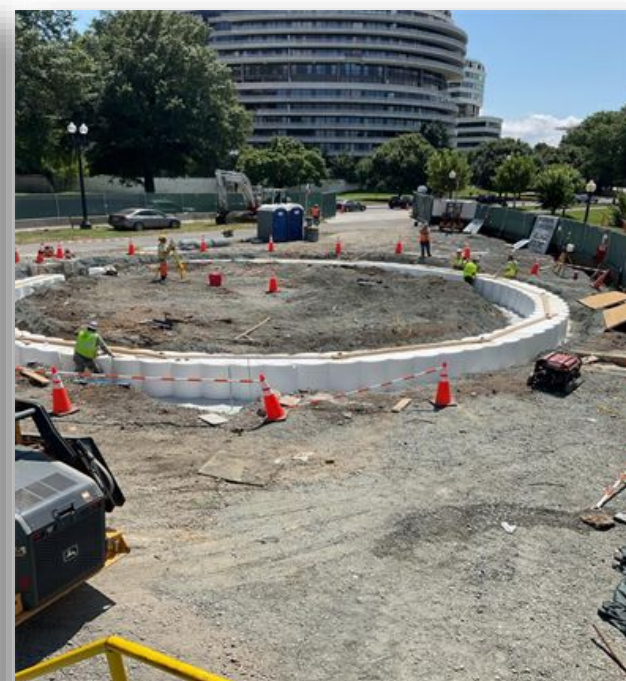
CSO 022 Installation of the Guide Walls for the Shaft
