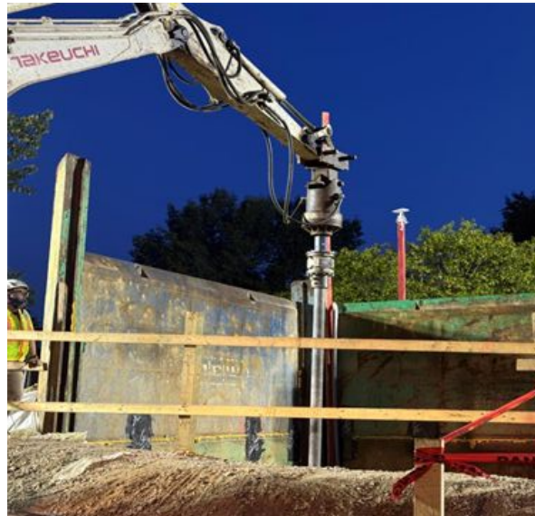
Helical Pile Installation
