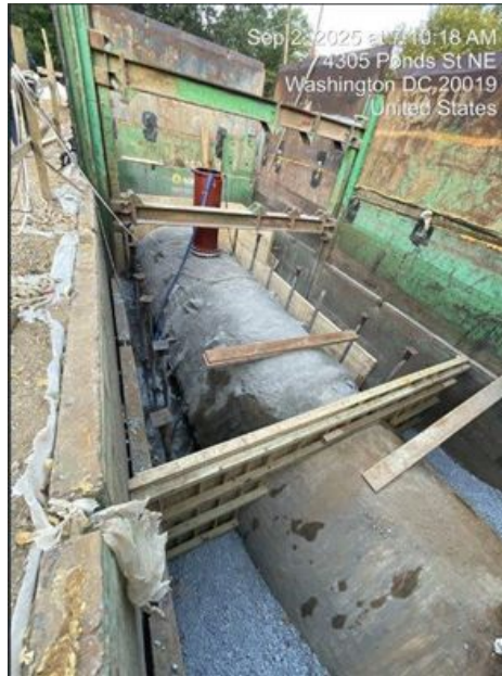
Installation of rebar and formwork
