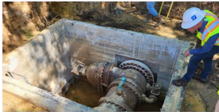
36" Valve Inspection at Fessenden Avenue NW
