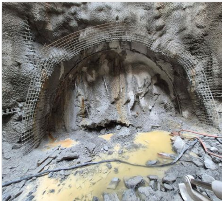
WPP Overflow Mining Shaft Starter Tunnel North
