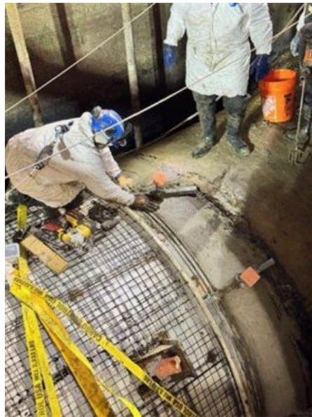
Infilling pipe gap with cement
