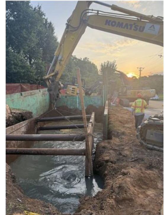
Shoring of the "pit"
