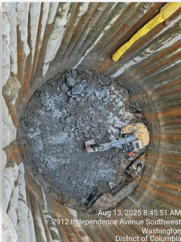
WPP Temporary Mining Shaft Rock Excavation
