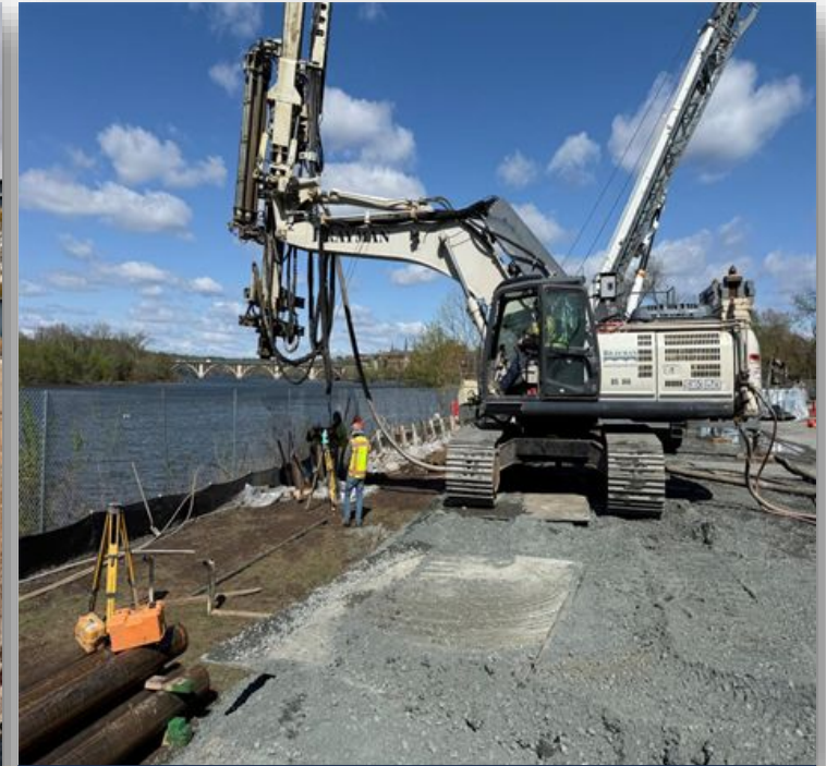
Installation of Micropile System to Protect Seawall during Construction
