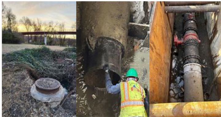
Pipe break on 30" pipe in Anacostia Park
