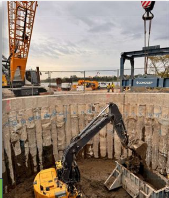
WPP Temporary Shaft Temporary Support of Excavation System
