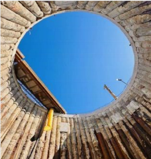
WPP Overflow and Mining Shaft Temporary Support of Excavation System
