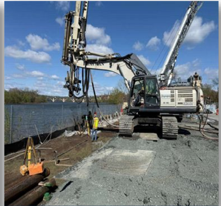
Installation of Micropile System to Protect Seawall during Construction
