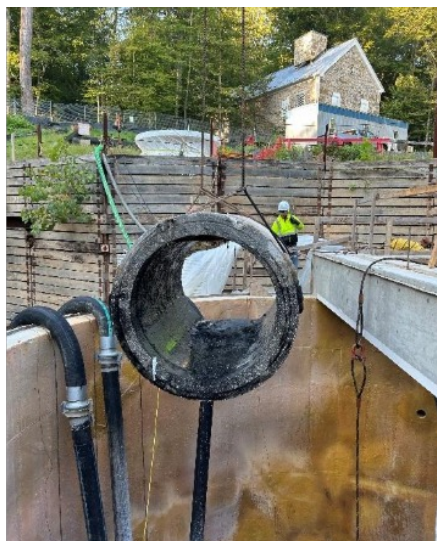
Removal of 54" RCP at MH-31
